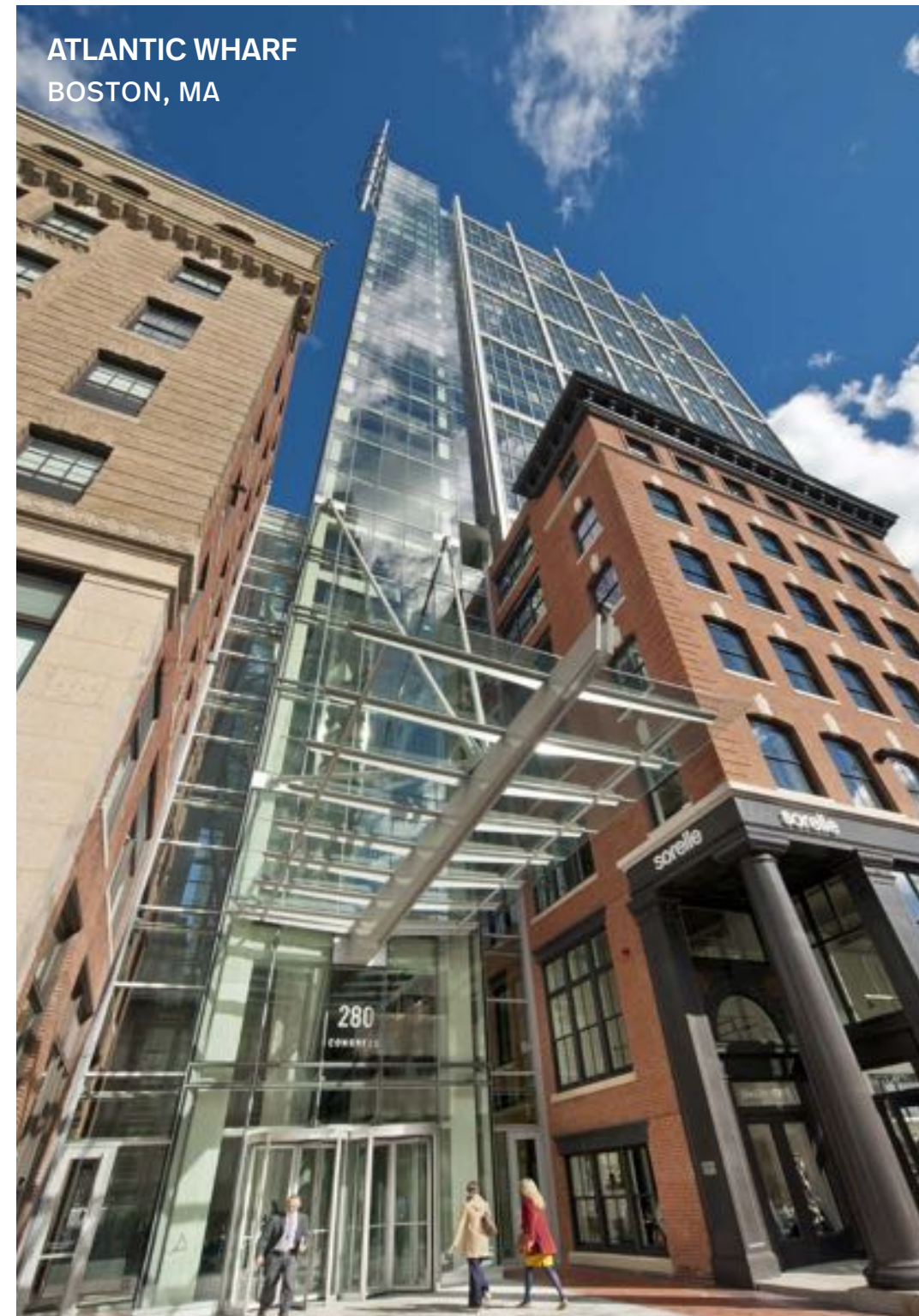
HARVESTING RAIN | Atlantic Wharf features a half-acre green roof that captures rainwater and has helped to save over 12.5 million gallons of water annually, equivalent to 19 Olympic-sized swimming pools.
