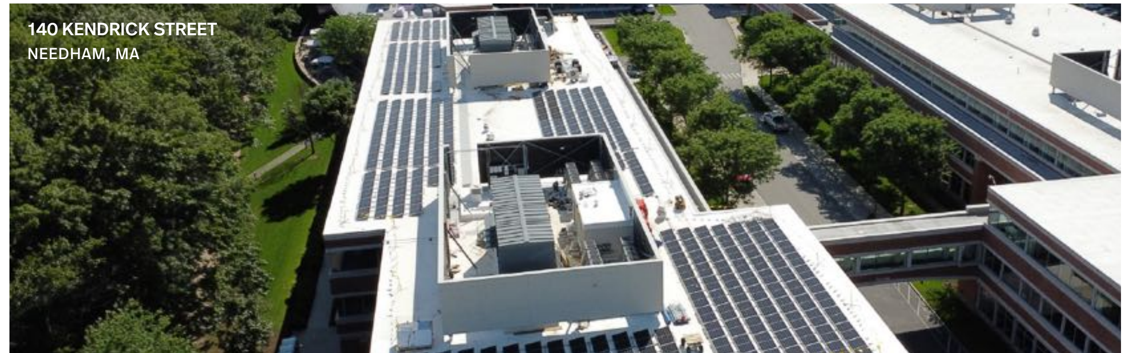
NET-ZERO DEVELOPMENT | BXP fully placed-in-service our first net-zero repositioning in 2023 at 140 Kendrick Street in Needham, MA. The scope of the renovation project included full electrification, building envelope improvements, advanced energy recovery systems, mechanical system modernization, and the addition of on-site renewable energy generation.
